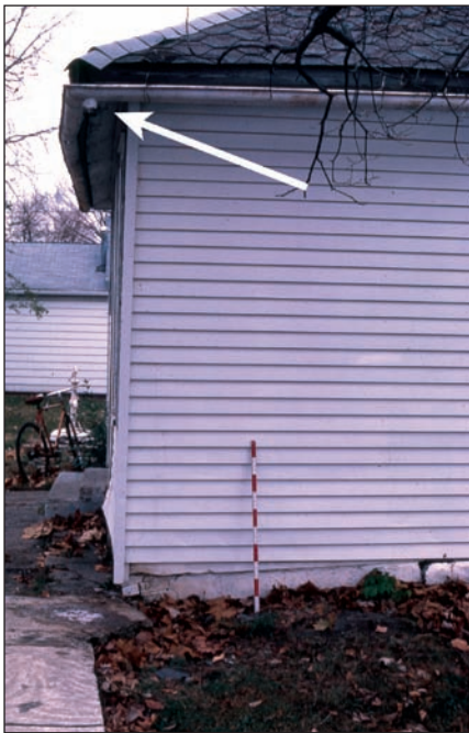
Figure 20 Foundation sinking at the corner of building due to reduced support caused by excessive, repeated moisture changes. Note gutter drainage (arrow) and lack of downspout to channel drainage away from foundation.
