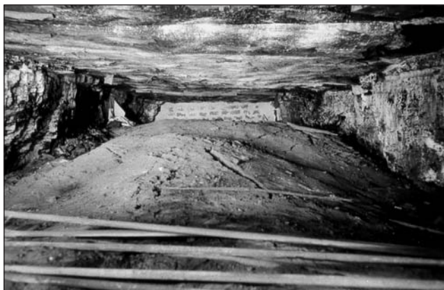
Figure 12 Diagram and photographs of coal pillars being pushed into a soft floor. The claystone material is being squeezed out from under the pillar up into the entryway.
